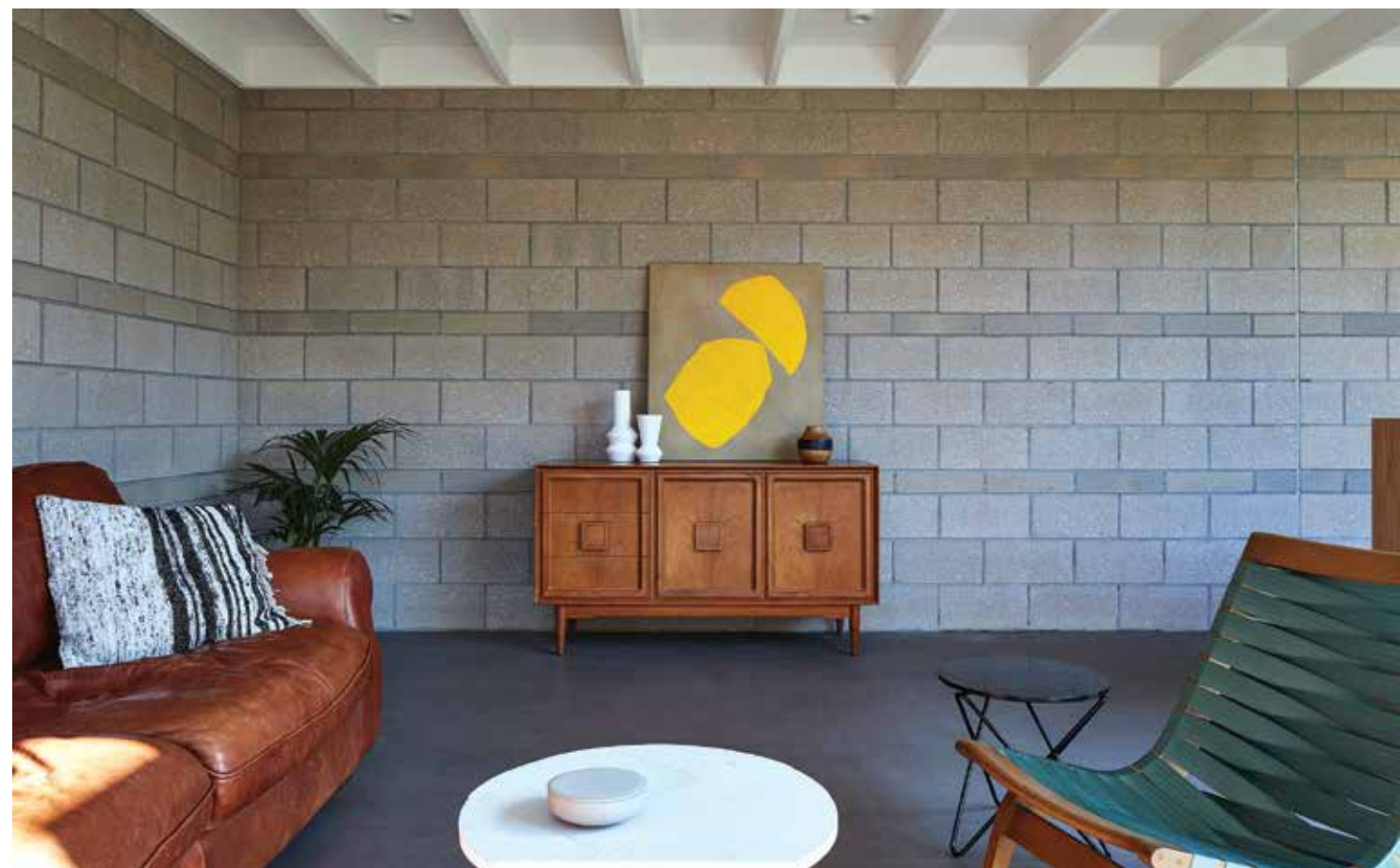
Winter sun warms the internal block walls providing thermal mass. opposite page The new internal boundary wall extends lengthways along the southern edge of the block.
